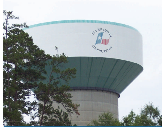
Water Storage Tank on Whitehouse Drive
