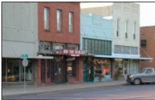
Illustration 10-19 An Example of a Downtown Area Without Visible Utility Lines
