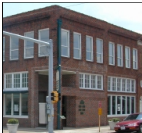
Illustration 10-24 Brick Materials on a Downtown Lufkin Building
