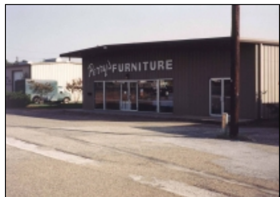
ILLUSTRATION 9-7: Example of Masonry and Metal Facades on Nonresidential Structures
