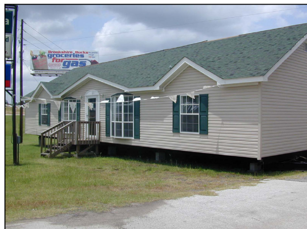
ILLUSTRATION 6-6 Example of a Manufactured Home With a 6:12 Pitched Roof
